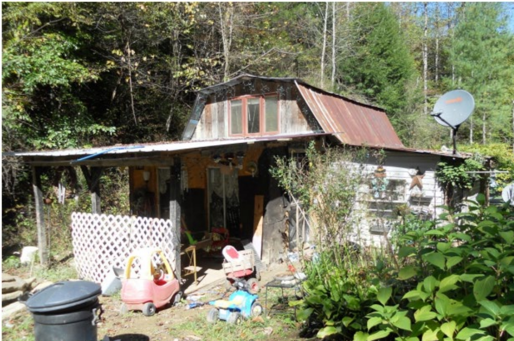
This house was originally built as a chicken coop. When the family had to move in, they added some rooms.
